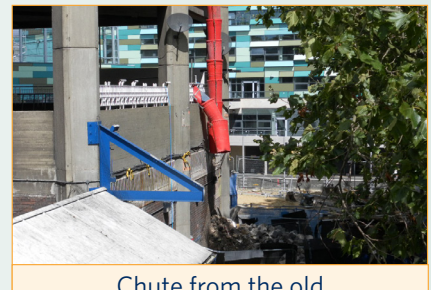
Chute from the old Social Services office
